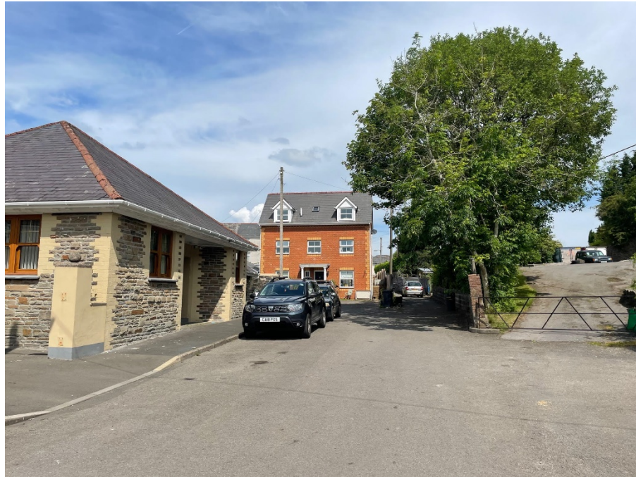
Fig. 1.1 Front Elevation of Existing Dwelling
